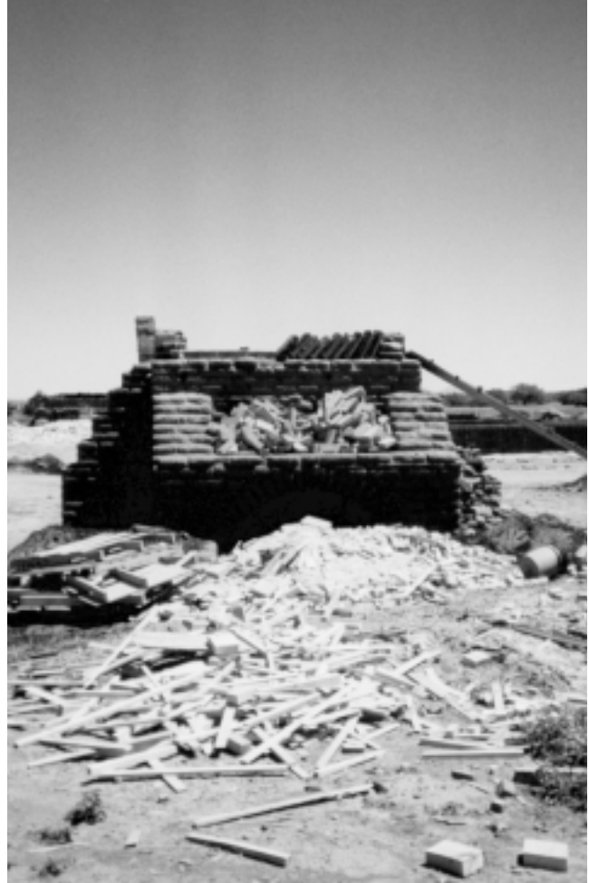
Typical traditional Mexican brick kiln.
