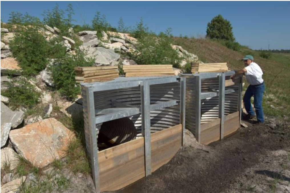
Rancher Jimmy Wohl inspects a berm and culverts with riser boards installed to retain water at Rafter T. Credit: E. Boughton/MAERC.
