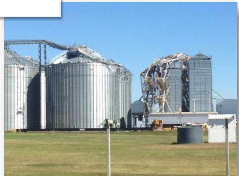
Storm Damage to (New) Grain Storage Facility [Dolores, 2013]
